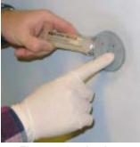
Figure 5-25. Apply rust inhibitor
