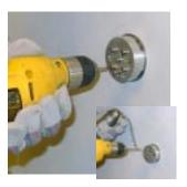
Figure 5-21. Drill Mounting Holes
